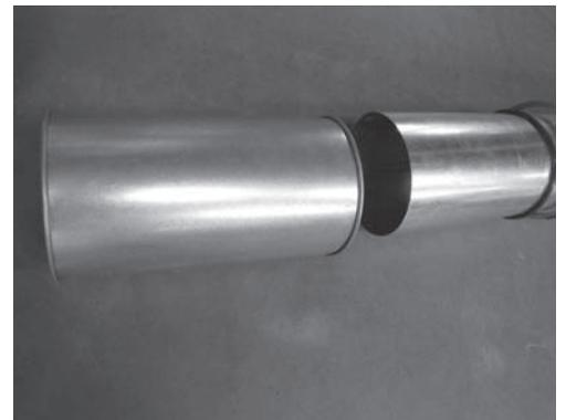
**Step 6.** Clamp ends of assembly. Clamp O-ring to sleeve.
